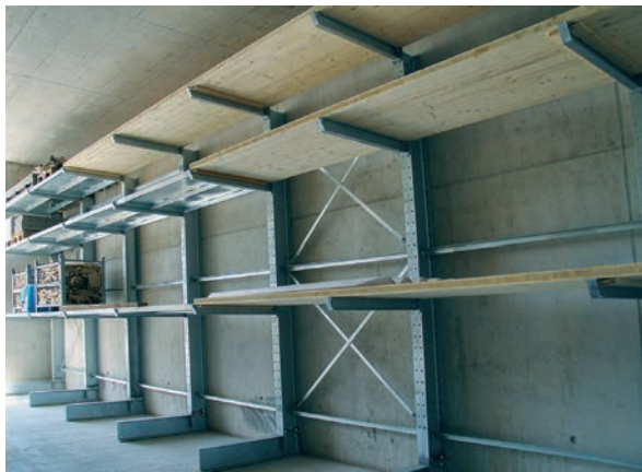
3 Cross-braces and horizontal braces for a secure bond
